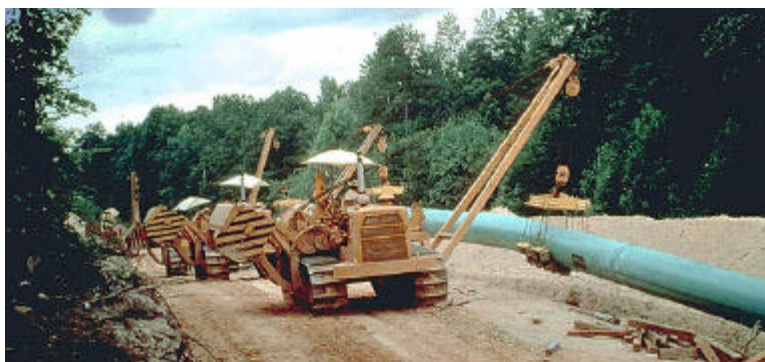
Figure 1. FBE coatings have been in use for underground and undersea pipeline protection for nearly forty years.
