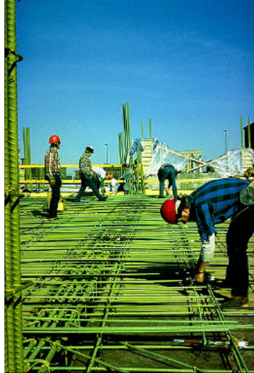
Figure 10. FBE coated rebar helps prevent corrosion and damage to concrete structures.
