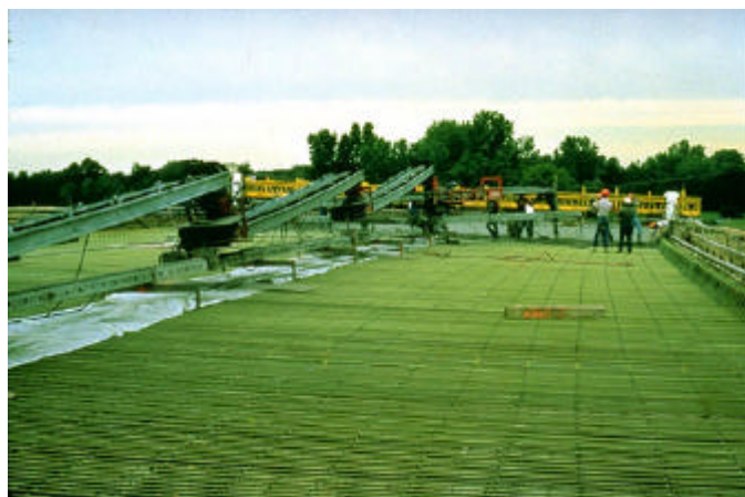
Figure 2. Specially designed FBE coatings on reinforcing steel have been installed in more than 100,000 structures in the US alone.
