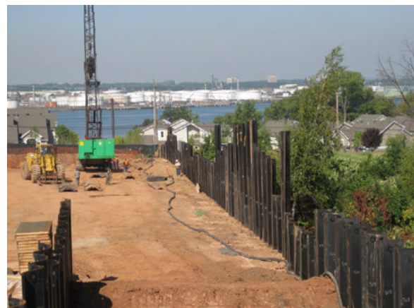
Elevated view shows construction of the foundation for the interior wall
