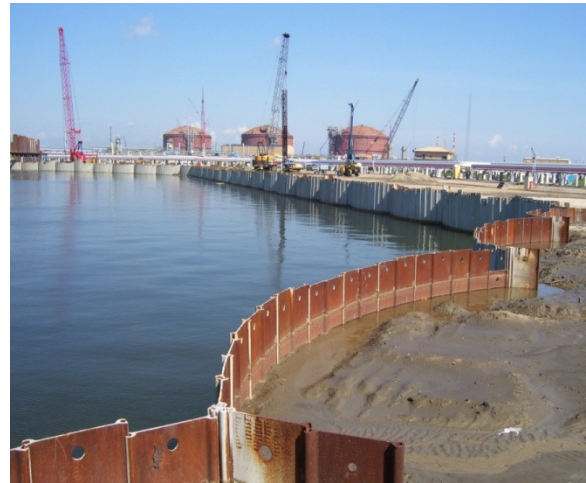
Ground level view of OPEN CELL structures
