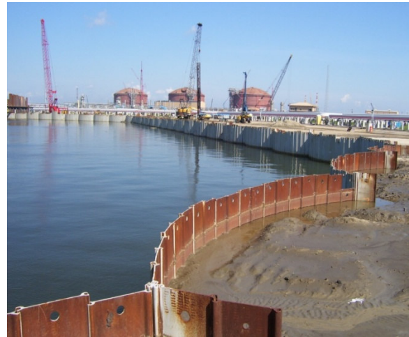
Ground level view of OPEN CELL structures
