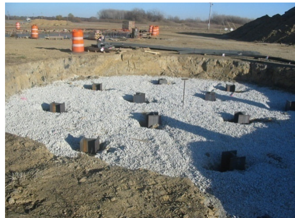
Driven piles before concrete cap is poured
