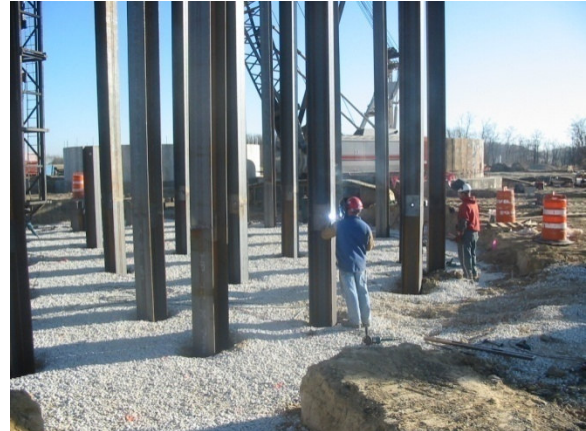
50 ft. H-Beam being spliced to 70 ft. H-Beam
