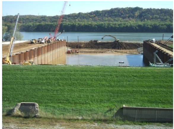
Ground level view of OPEN CELL structure
