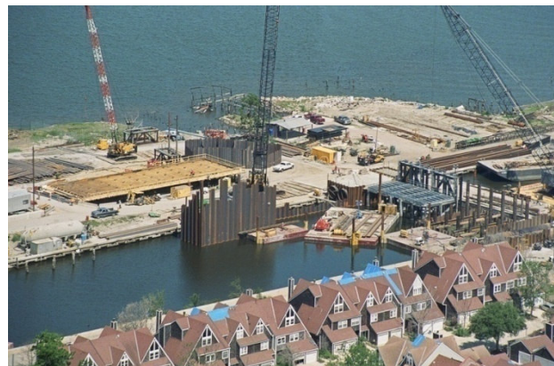
Sheet piles driven around perimeter of foundation. The sheet pile functioned as a cutoff wall and as a cofferdam.
